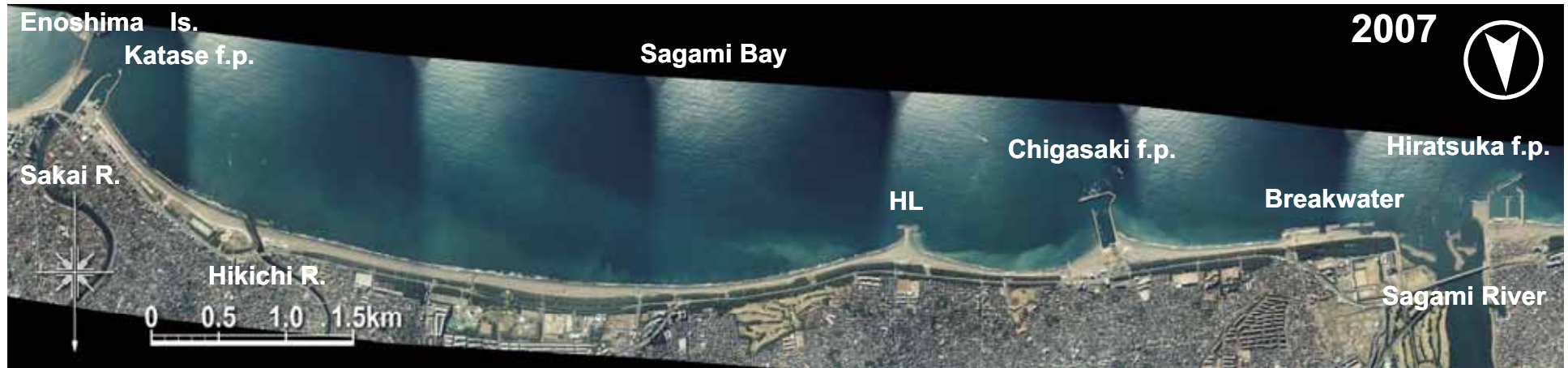
Aerial photograph taken between 1954 and 2007.
